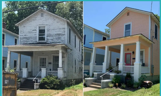
Figure 5: Example of a rehabilitation of a home.
