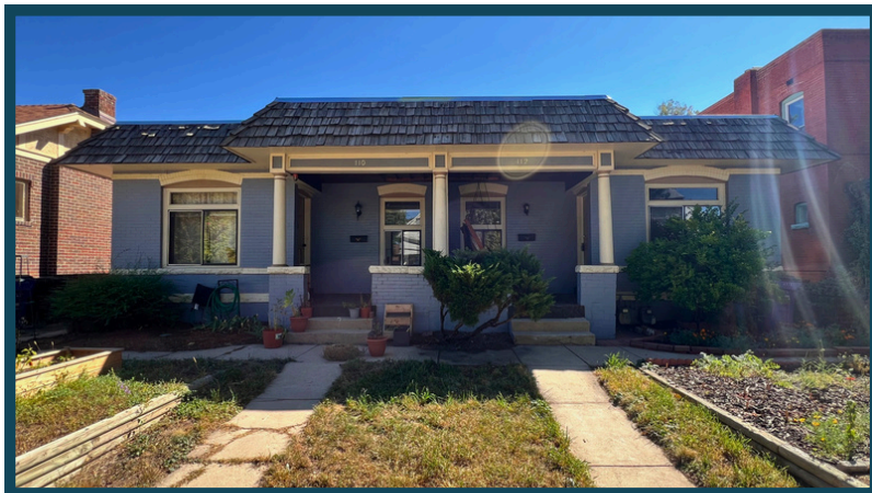
Side-by-Side Duplex in Denver. Source: C. Noto
